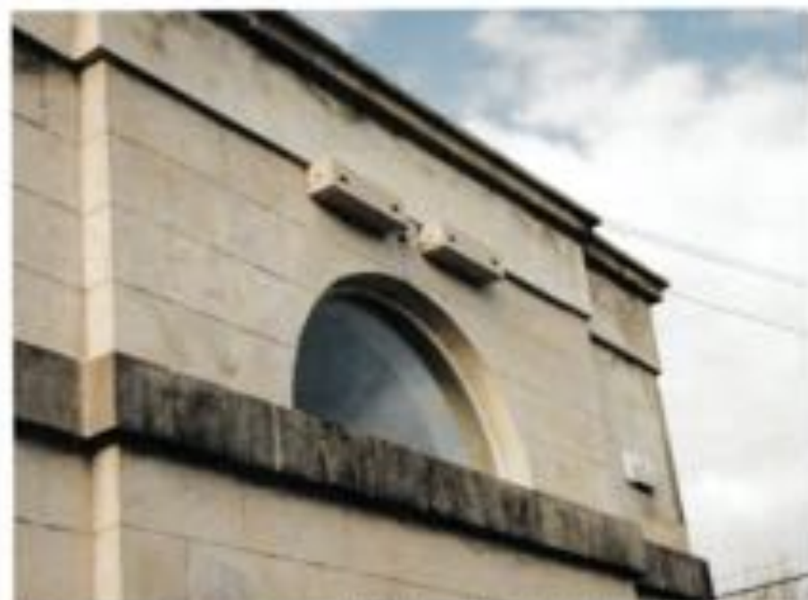
Swift boxes, consisting of nest sites, installed on the side wall of the Dughterard Courthouse.
