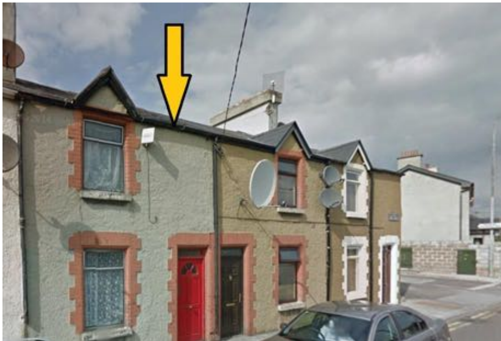
No. 18 Urban Terrace. Orientation is South East
