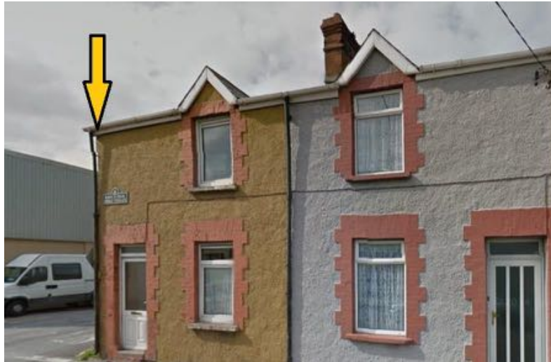
No. 1 Urban Terrace. Orientation is South East
