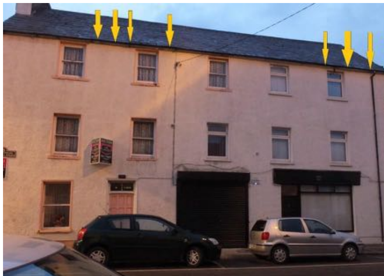
Front of the building on Pembroke Street. Orientation is South West
