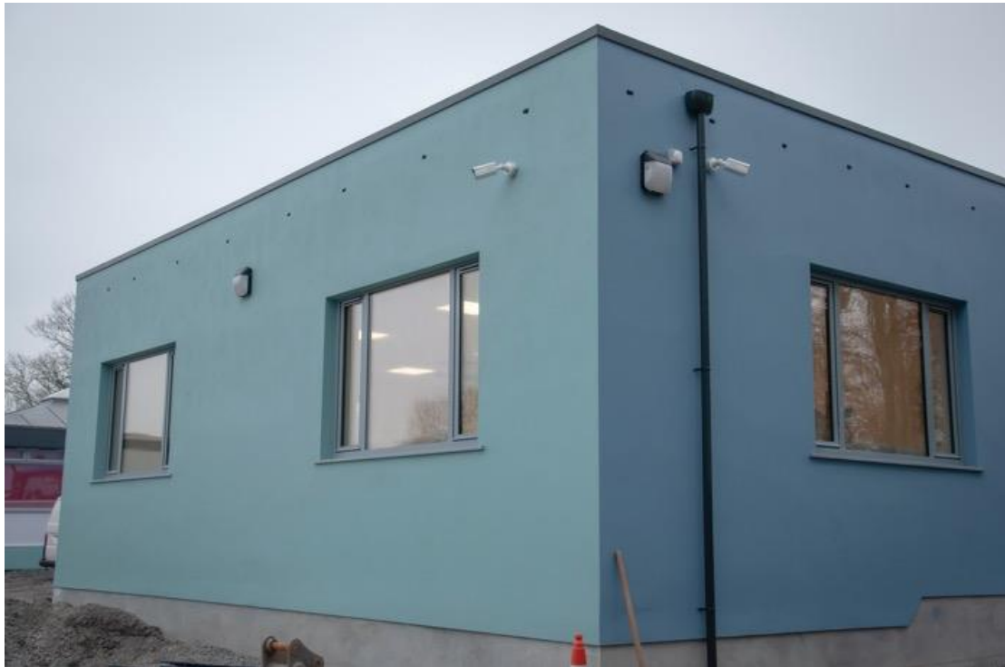
Picture 8. Ballinrobe National School pool wall finished with nest box entrance holes clearly visible in a horizontal row.
