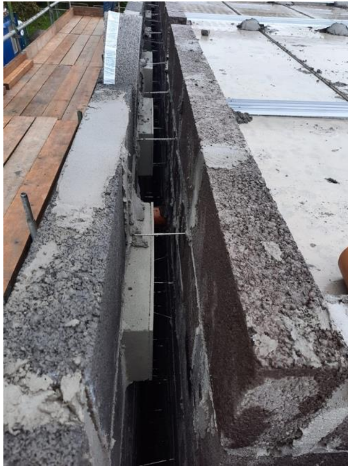
Picture 5b. Woodstone nest boxes incorporated in walls of Ballinrobe NS, Co. Mayo
