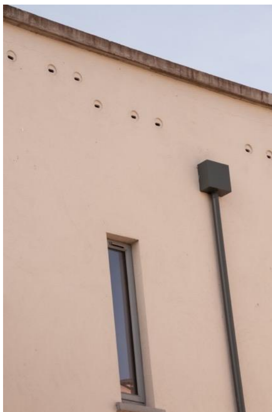
Picture 1. Westport Town Hall built-in boxes in June 2018 - no marks of bird droppings on the wall.
