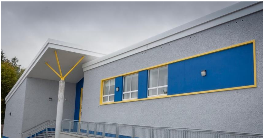
Picture 9. Mount St Michael project completed with entrances aligned and call system in place
