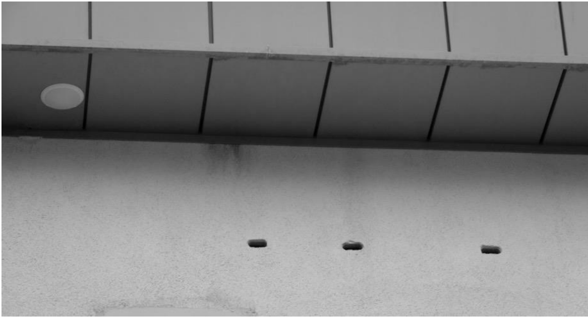
Picture 10. Sancta Maria College in Louisburgh will speaker installed in soffit above nest boxes
