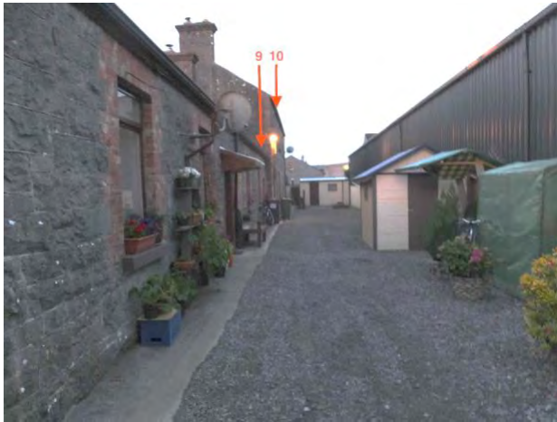
Rear of Old Station House facing SW
