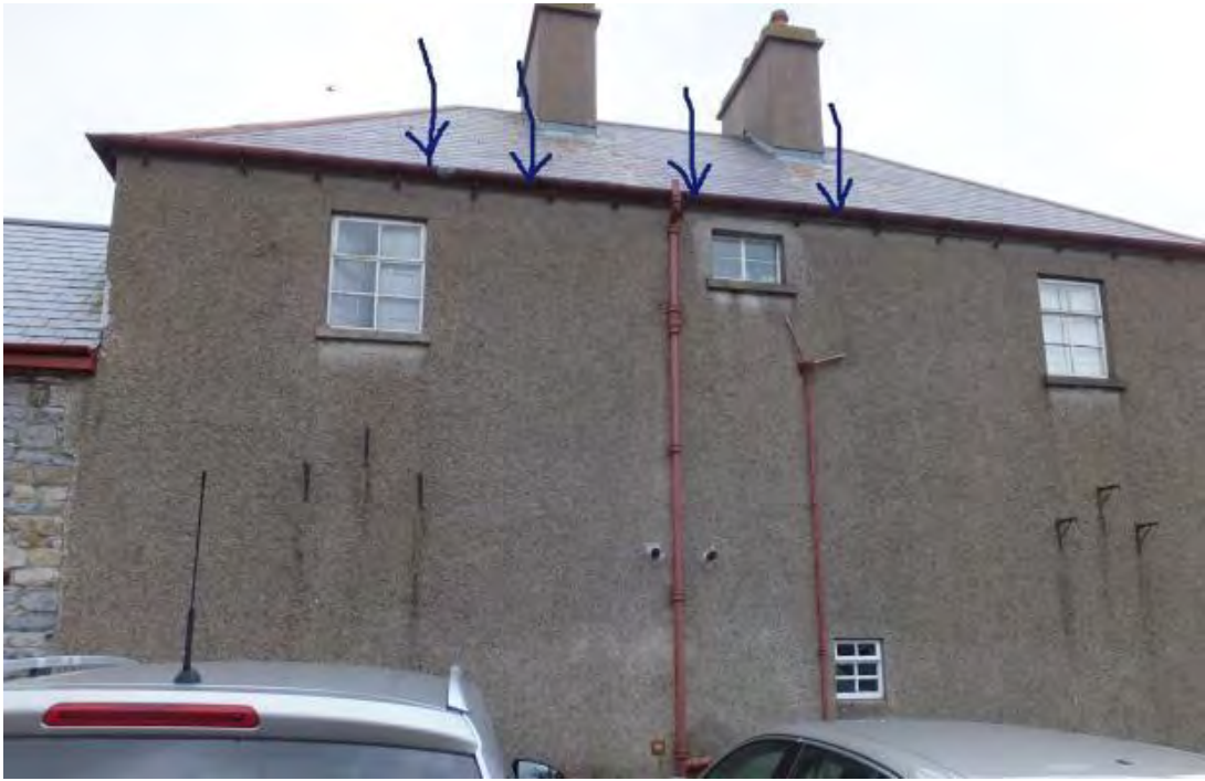
Rear of building facing west
