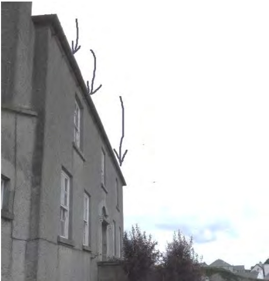
Front of building facing east
