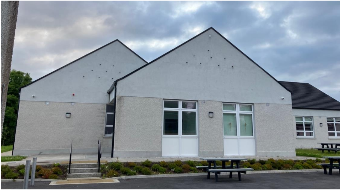
1b. Two gables each with 8 built-in GZ03 nest boxes – entrances are staggered
