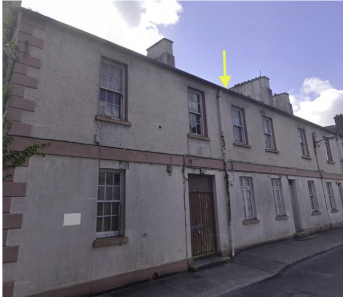
2c. NE - 2024 there was only one nest active near area of fire on left side of building (see 1a and 1b)
