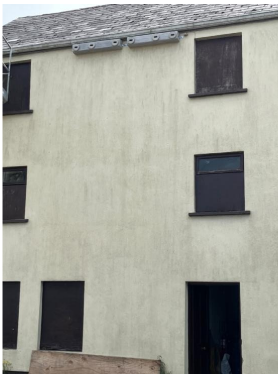
18a. Two Schwegler 17A nest boxes installed by IFI in July 2024
