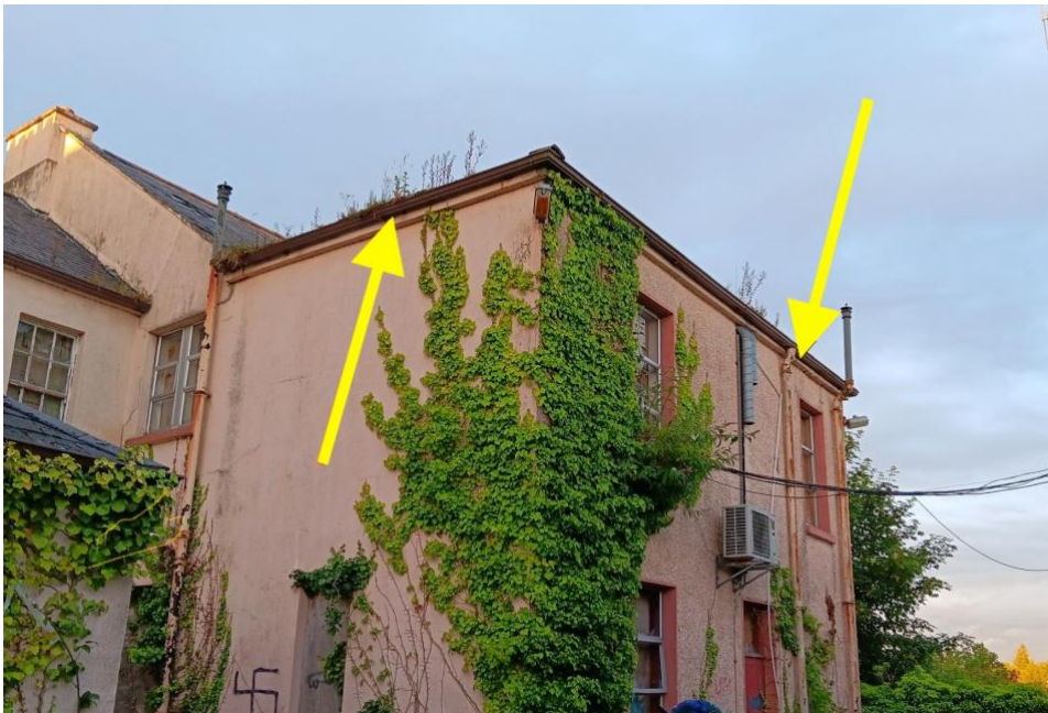
2f. SW - Rear of building
