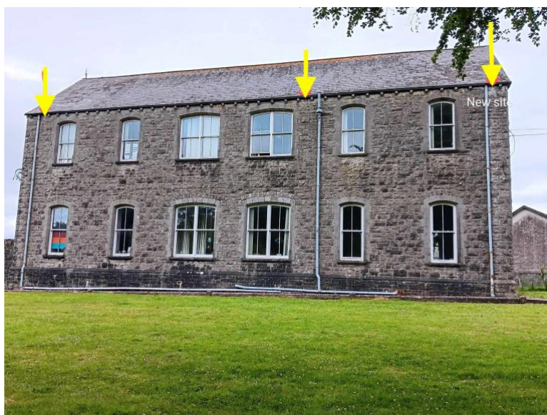
10a. NE side of building
