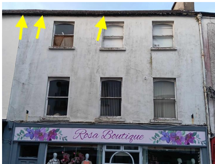
5a. SW facing on Lower Tone Street
