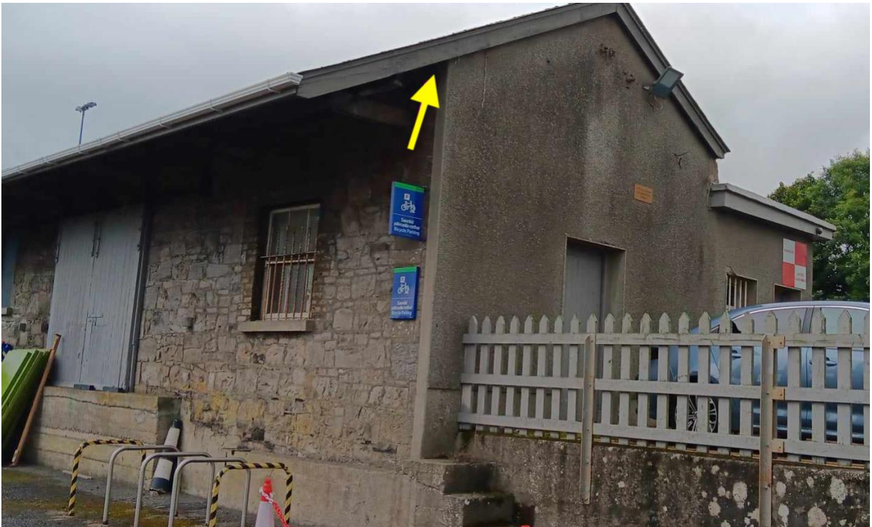
1d. East facing at edge of canopy
