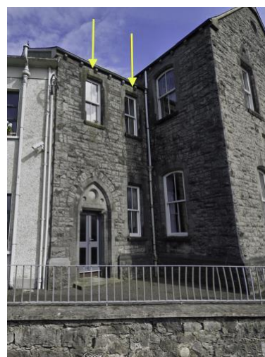
10b. SE front of building
