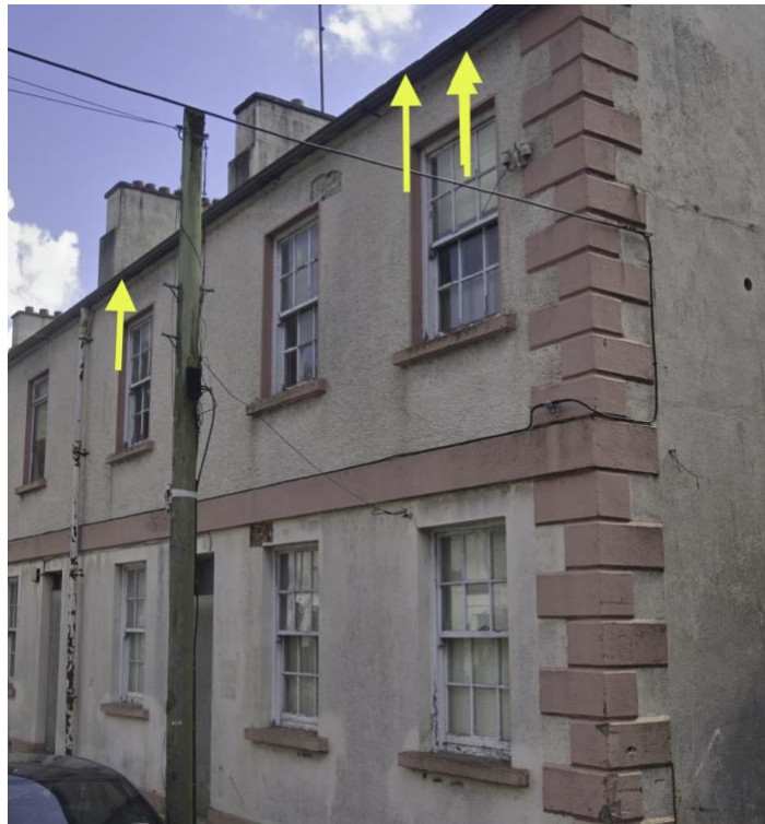
2d. NE - Right hand side of front of building
