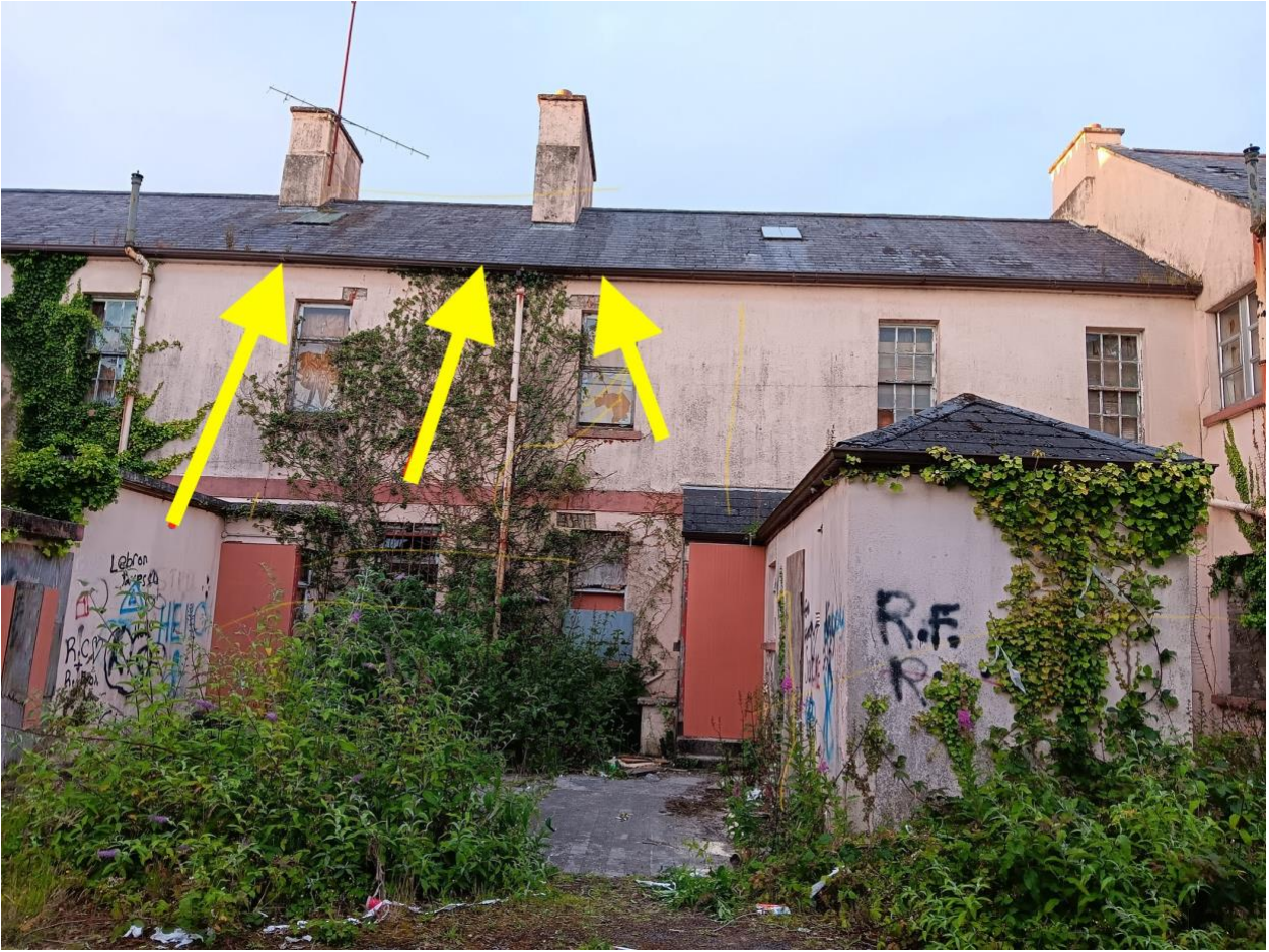
2g SW - Rear of building
