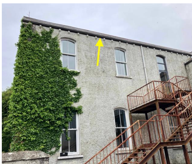
10c. NW at rear of building
