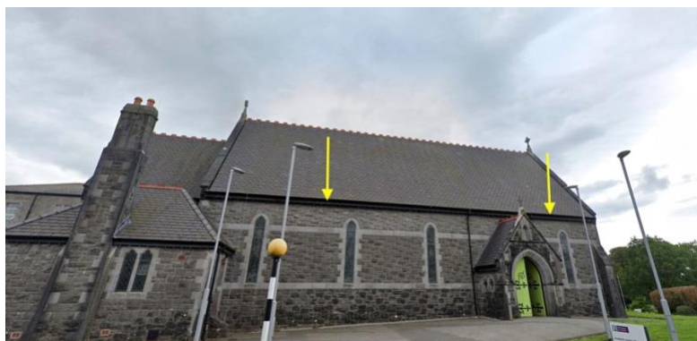
4b. North facing with two nest sites occupied. The nest site on the left is a new site whilst that on the right is one of the original nest sites preserved during building renovation.
