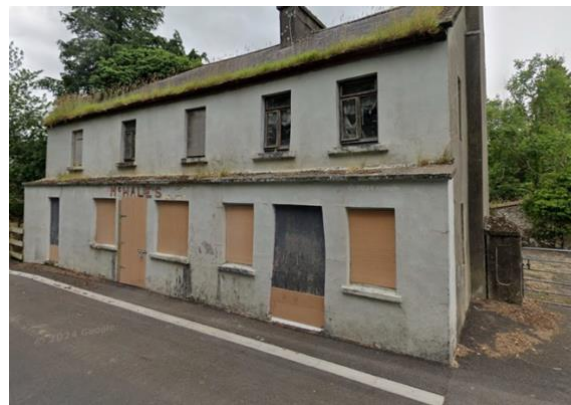
1a. Front of building – no nest sites observed
