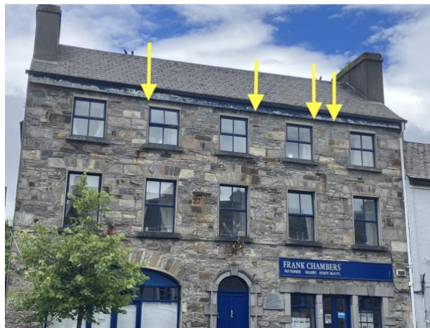
2a. West facing onto Main Street
