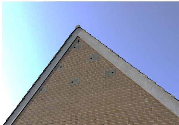
1a. South East facing – 6 built in GZ03 nest boxes.
