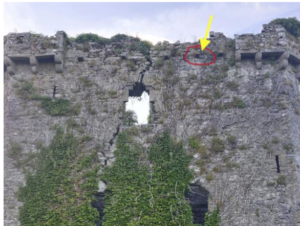
1d. South face – close up view of nest location
