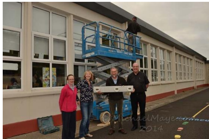
3a. 2014 – 2 x Schwegler 17A installed
