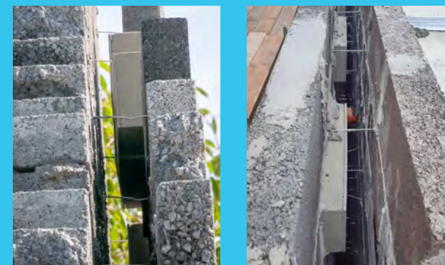
PICTURE 5. The nest box protrudes a few centimetres into the cavity but there is room for insulation
