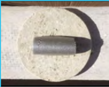
PICTURE 15. Nest entrance hole protected with piece of foam prior to rendering
