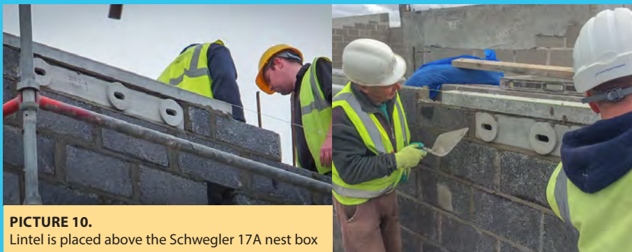
PICTURE 9. The nest boxes can easily be incorporated into a block wall
