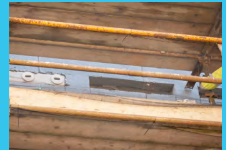
PICTURE 13B. The nest box was slotted into the space and secured with adhesive.
