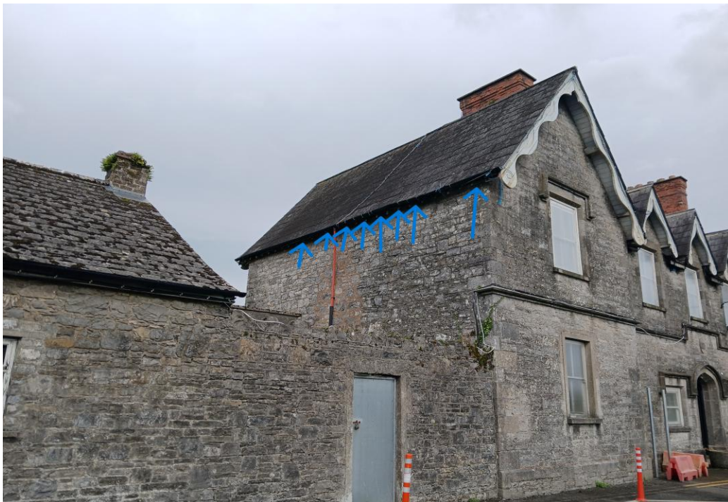
2a: Front of building (8 nests)
