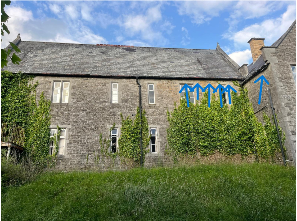
1d: Left side of building (6 nests)
