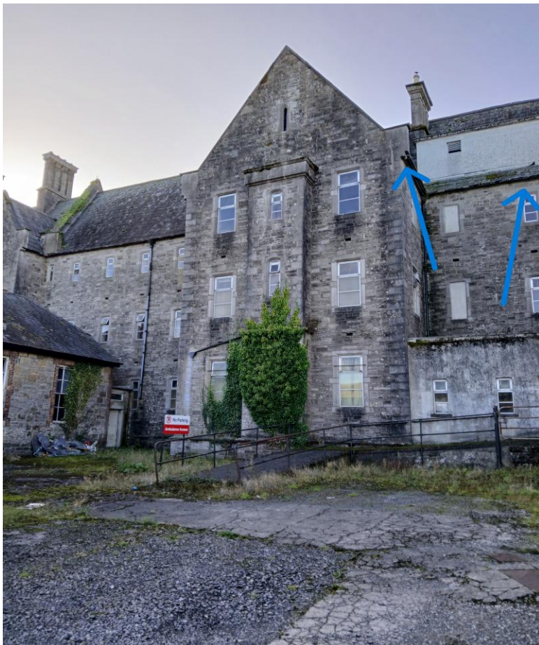
1j: Rear of building (2 nests)
