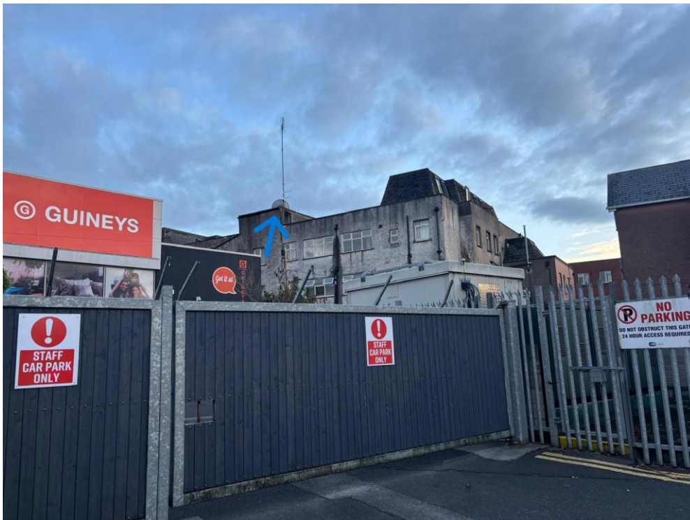
10a: Rear of building (1 nest)
