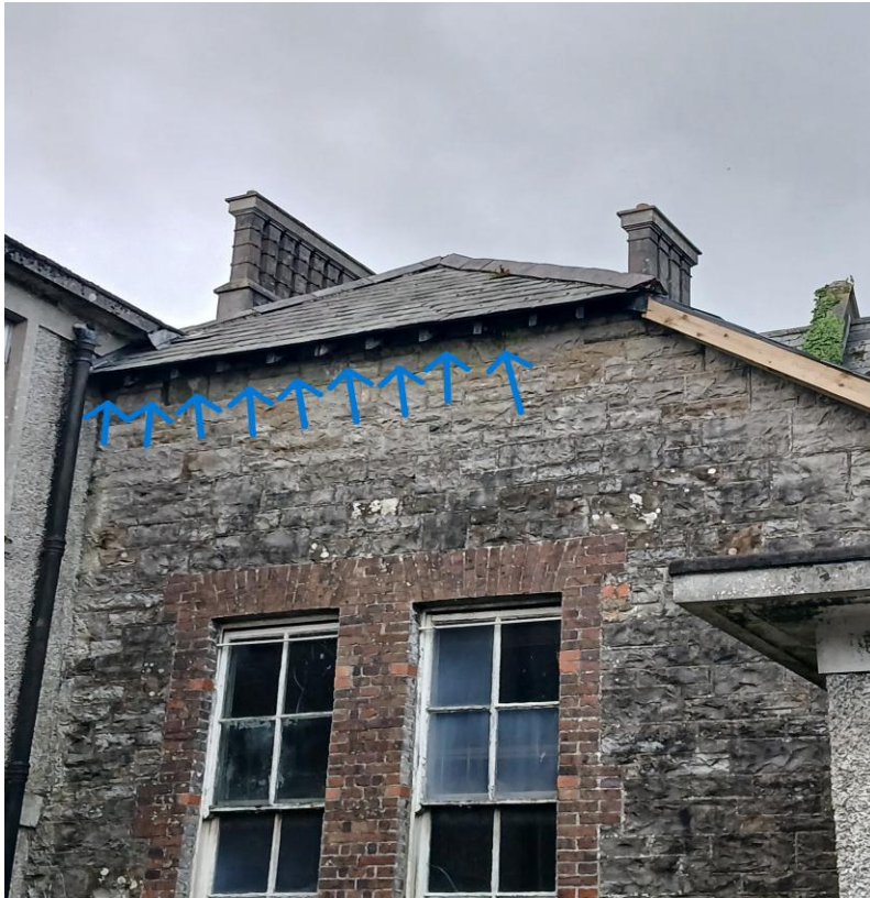
1k: Rear of building (9 nests)
