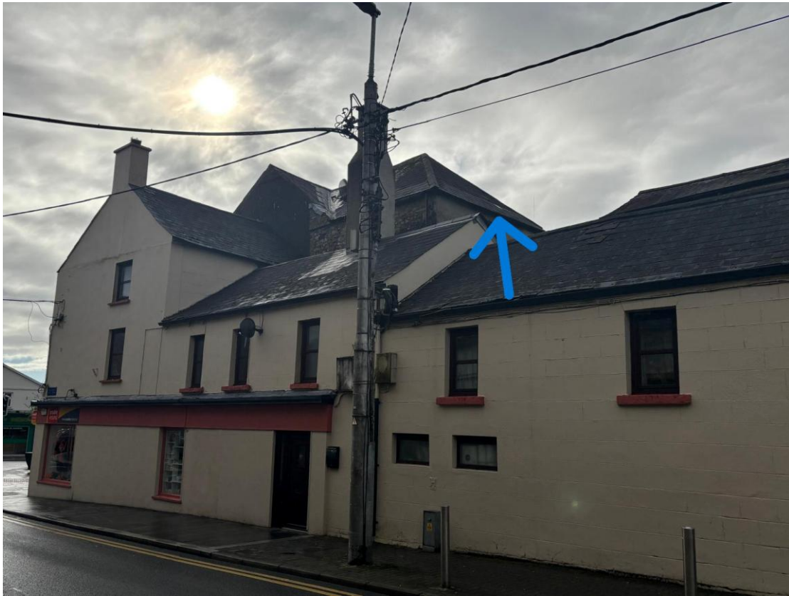
11a: Rear of Building
