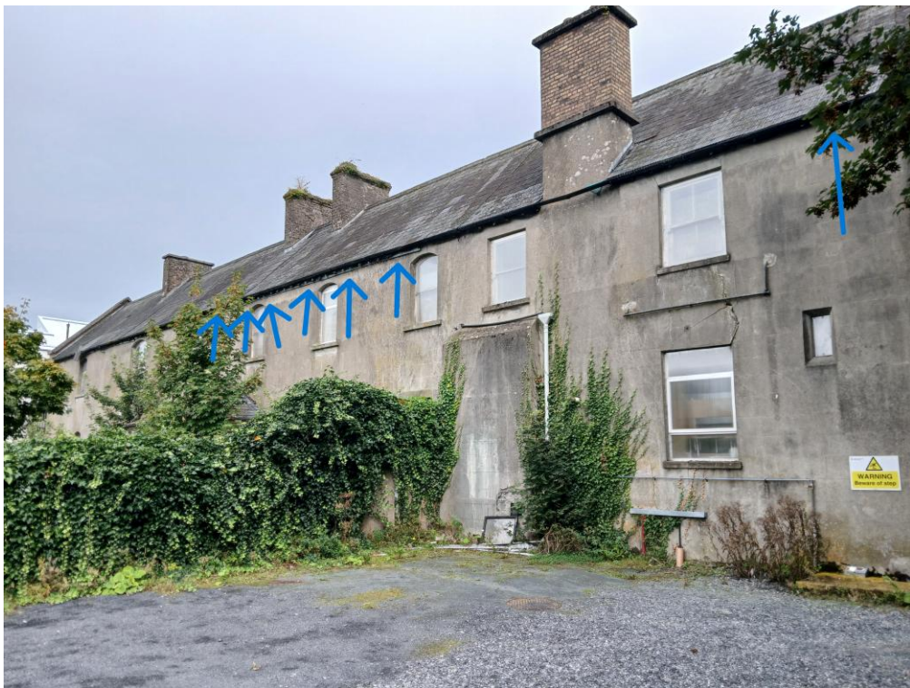
2c: Left side of building (7 nests)
