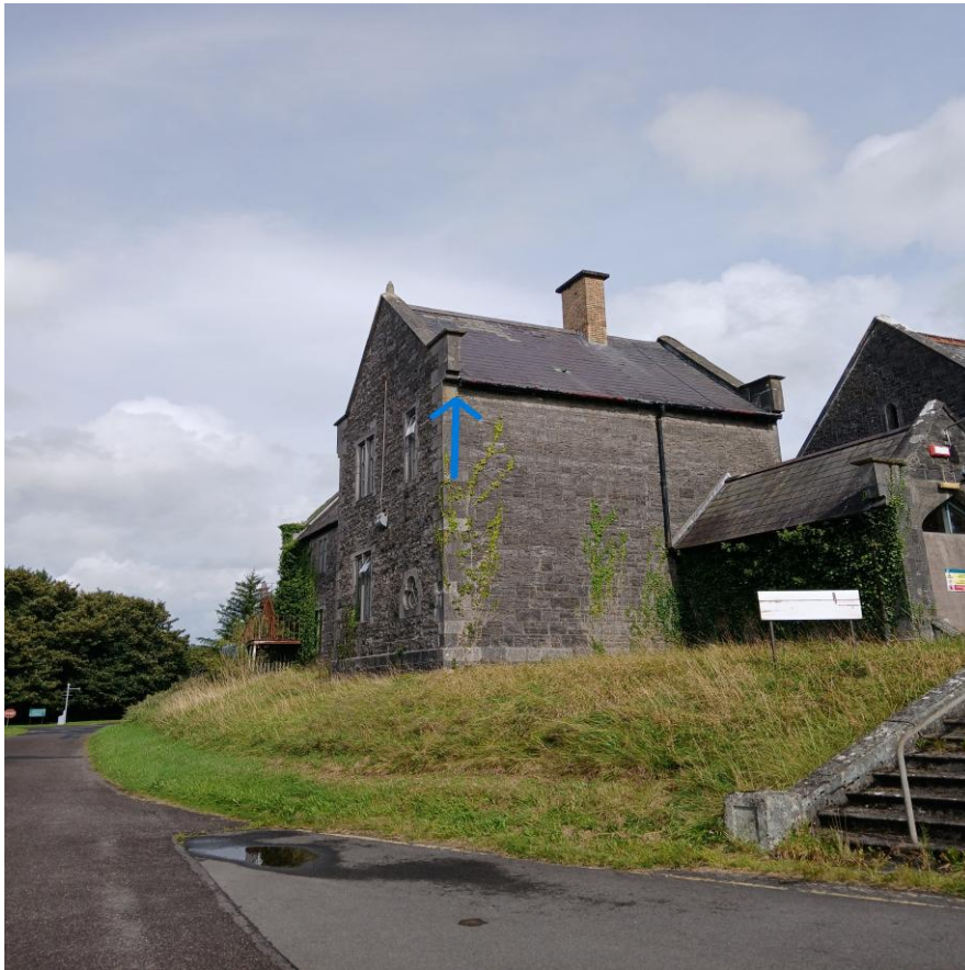
1c: Left side of building (1 nest)
