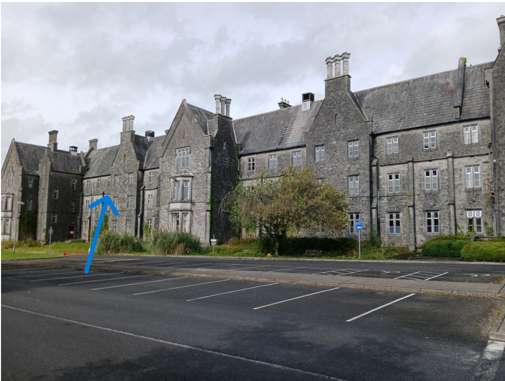
1b: Front of building, left hand side of main entrance. (1 nest)
