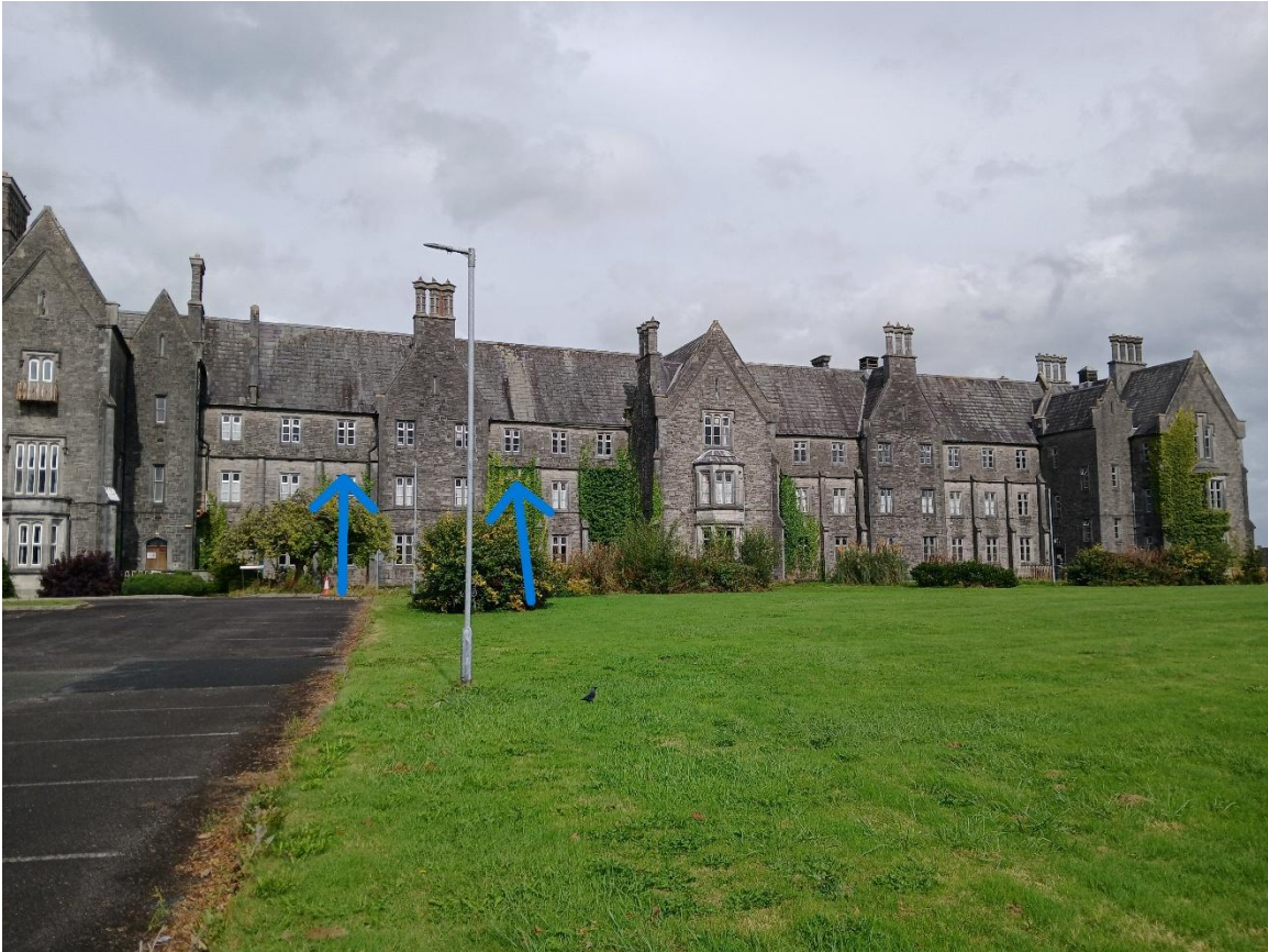
1a: Front of building, right hand side of main entrance. (2 nests)
