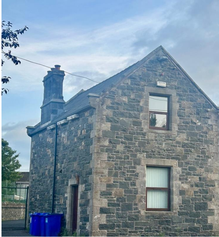
Model School – 2 additional boxes fitted
